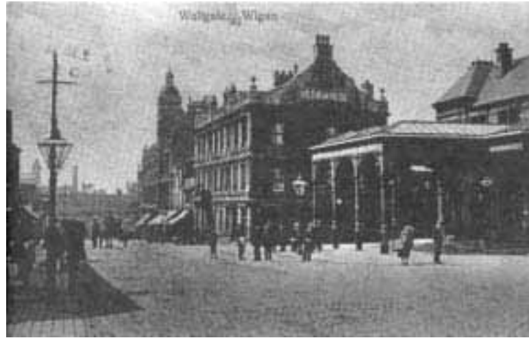
Wallgate c.1900 - note Wallgate Station, the Victoria Hotel and Tower Buildings.
